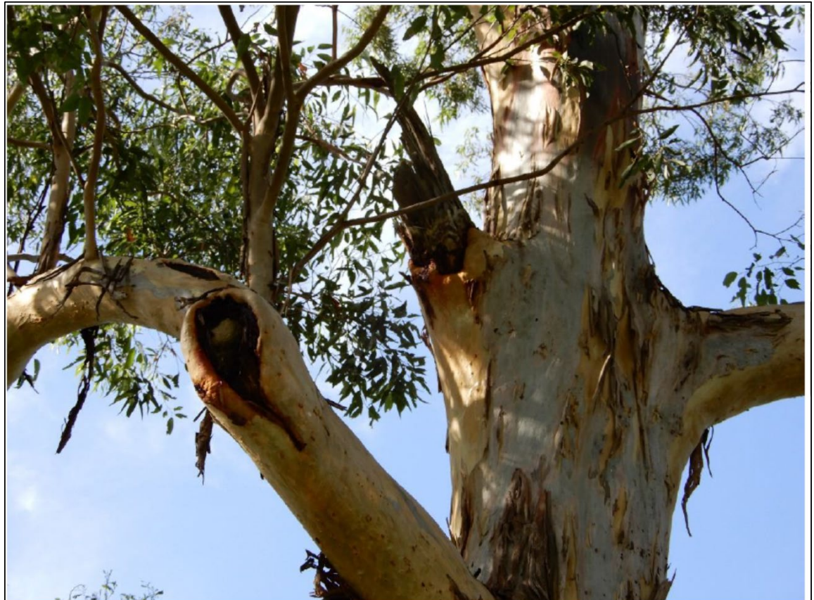
Photograph 6: Illustrating past branch failures – tree 10.
